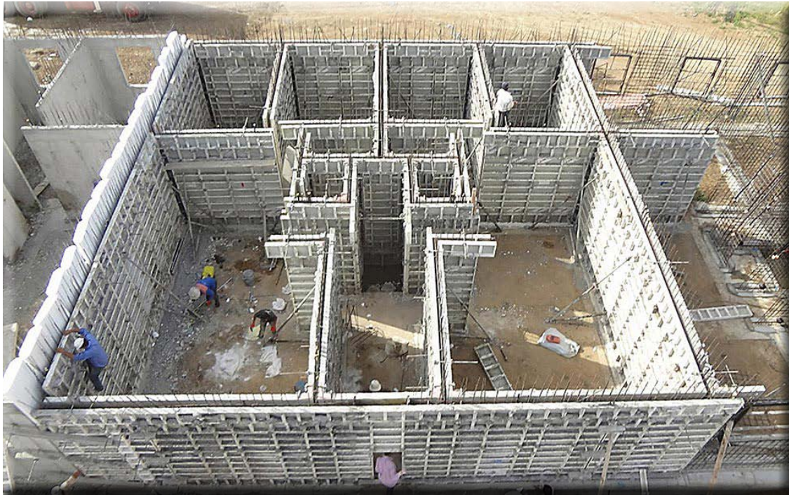
Practical application of aluminium formwork system
