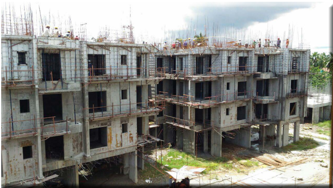
Construction site of aluminum formwork system
