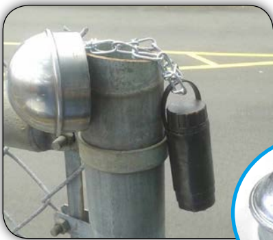
Dome-shape post cap covers on post
