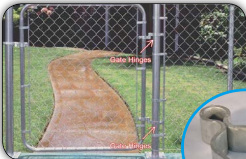
Gate frame hinge tightens post and panel
