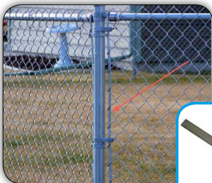
Tension bar attaches chain link panel
