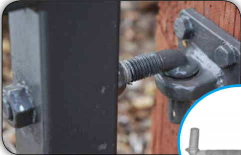
J-bolt hinge connects post to the wall
