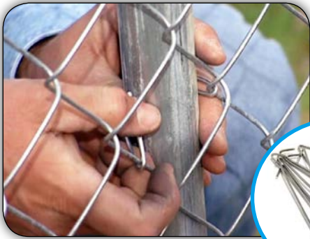
Application of fence ties
