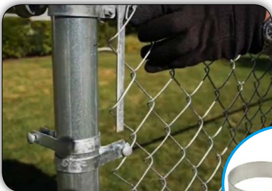
Tension band reinforces chain link fence
