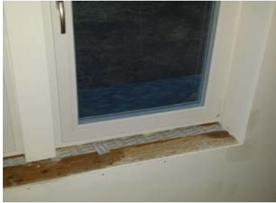
Finishing the seams of walls and windows.
