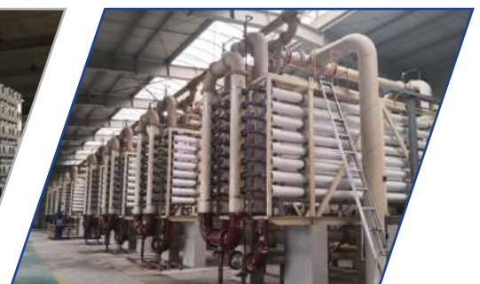
Dalian Hengli petrochemical water treatment project. Nov 2017
