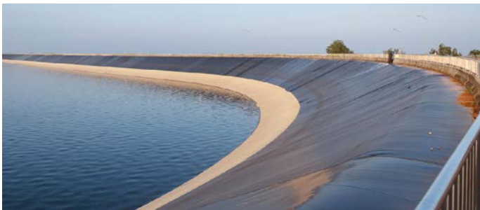
Geomembrane in embankment
