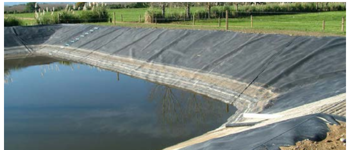
Geomembrane in artificial lake
