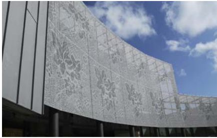
Perforated metal building facades.
