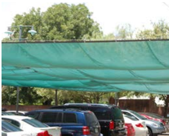
Horizontal debris netting parking lot.
