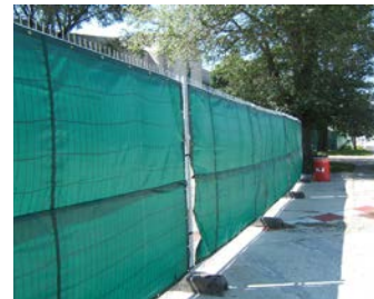
Vertical debris net road isolation.
