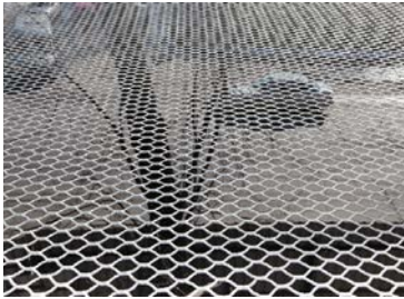
Horizontal debris netting one layer.
