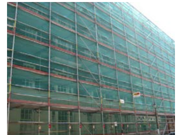
Vertical debris net construction.
